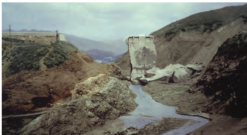
Fig. 4. The remains of the St Francis Dam after its catastrophic failure, with only the narrow middle section, subsequently known as the tombstone, still standing. The landslide scars in the eastern abutment are devoid of any plant cover on the right. On the western abutment, on the left, the reddish ground of scoured conglomerate is separated by the fault outcrop from the lower grey slopes of scoured schist. The boundary with grass-covered slopes above marks the lower level of floodwater erosion due to the delayed failure of the western part of the dam.
